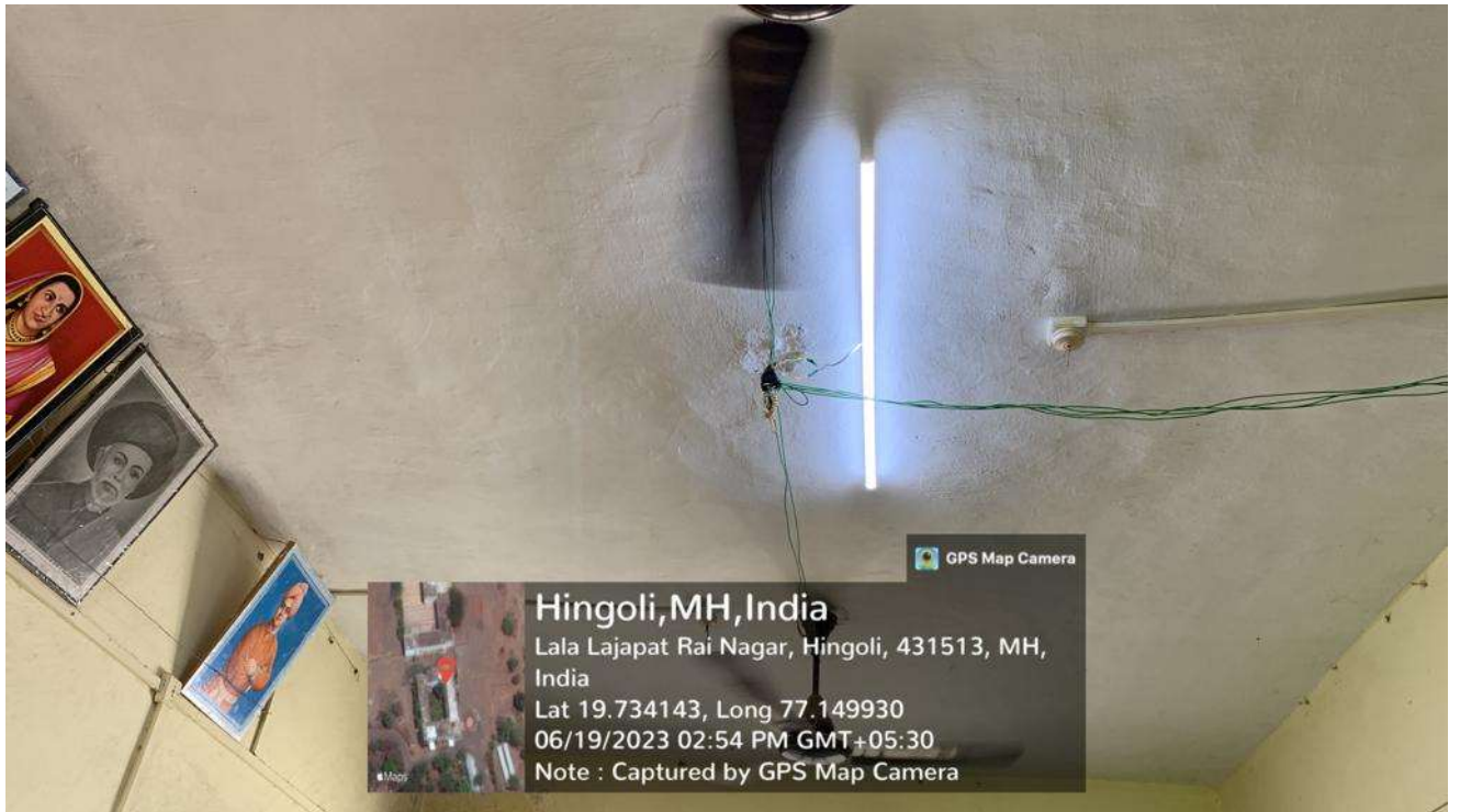
Use of LED in Vice Principal Office
